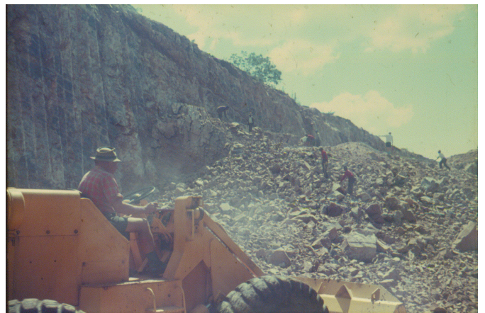
Removing the rubble & showing the 9:1 rock face.
